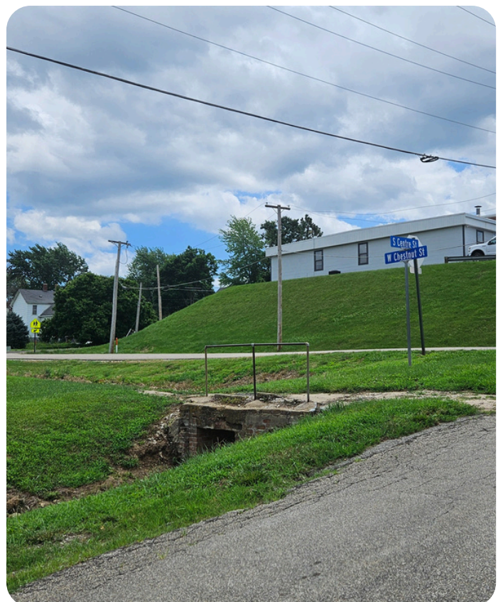
Culvert in Troy, KS
