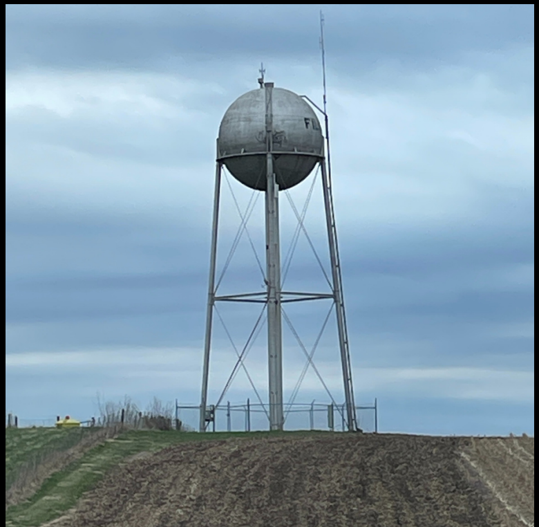
Water tower in Fillmore
