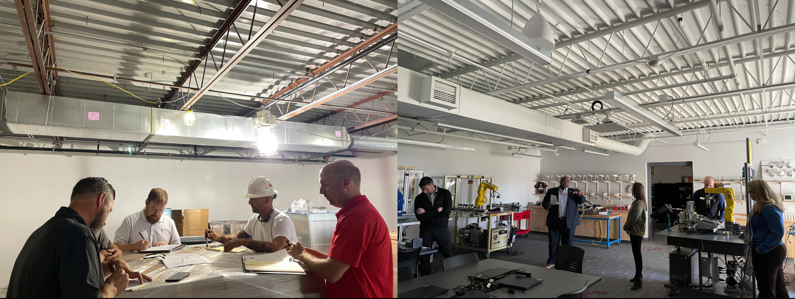
In progress to completed images of NCMC's remodel from McCarty Motors to robotics lab
