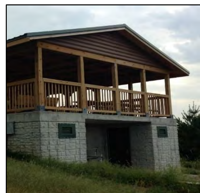
Image of Scout Camp Geiger Tornado Shelter
