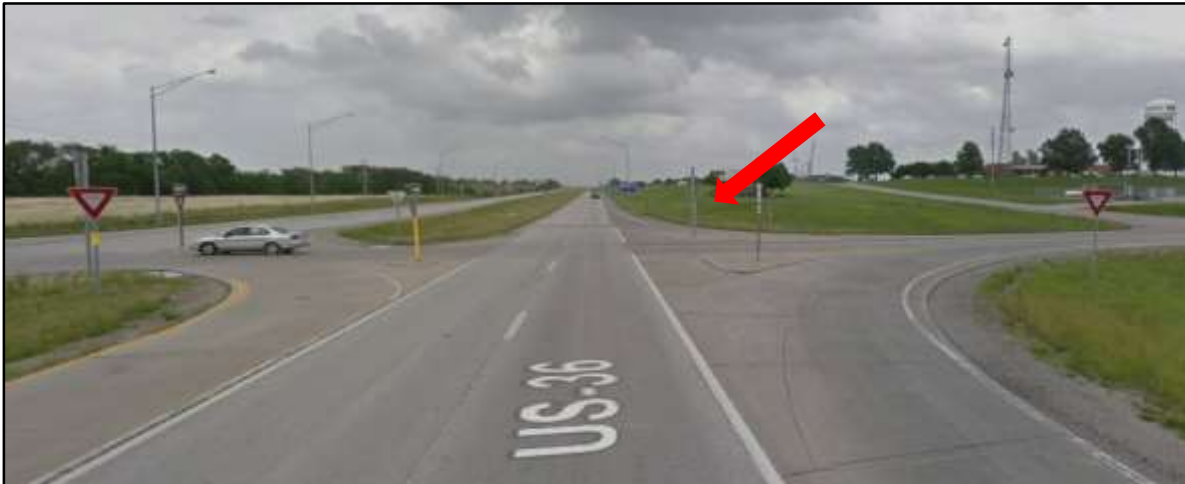
Figure 9 – View of Eastbound US Highway 36 at RSA location
