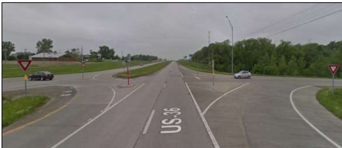
Figure 8 – View of Westbound US Highway 36 at RSA location
