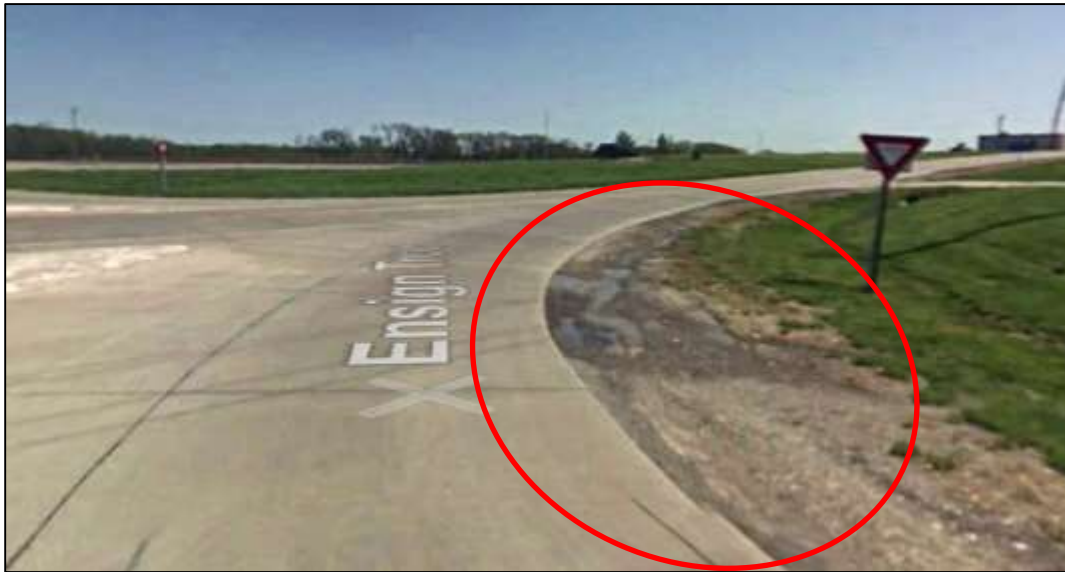
Figure 18 – Replace Gravel Shoulders with Concrete
